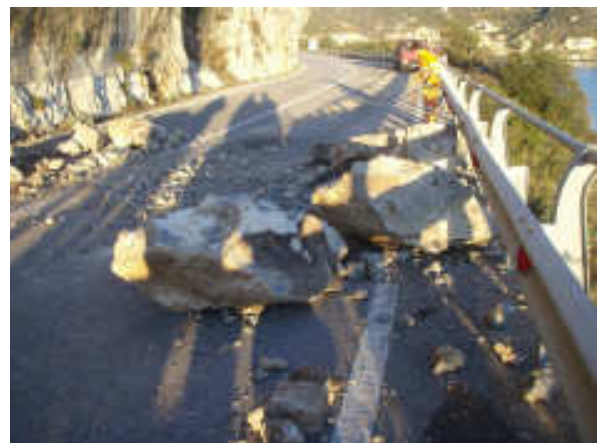
Fig. 3 – Rockfall affecting the Capo Noli cliffs on 16 January 2008.
